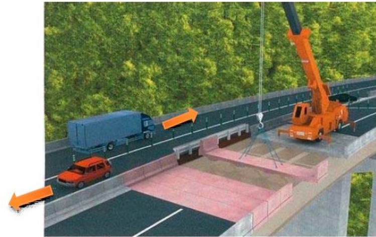
A crane moves deck slabs into place
